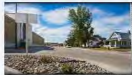
Wyoming/Park Area Phase 1 Complete
